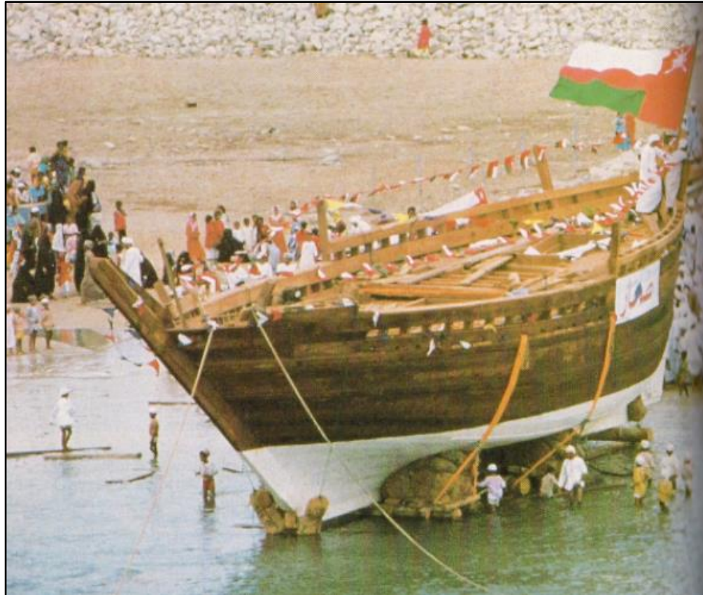
The launching of the hull
