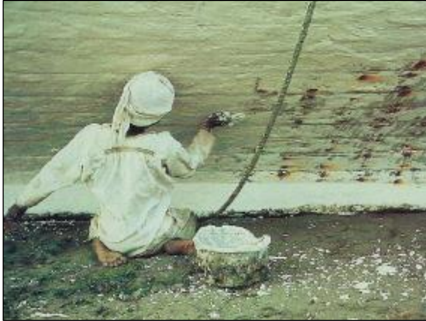
Applying the anti-fouling mixture
