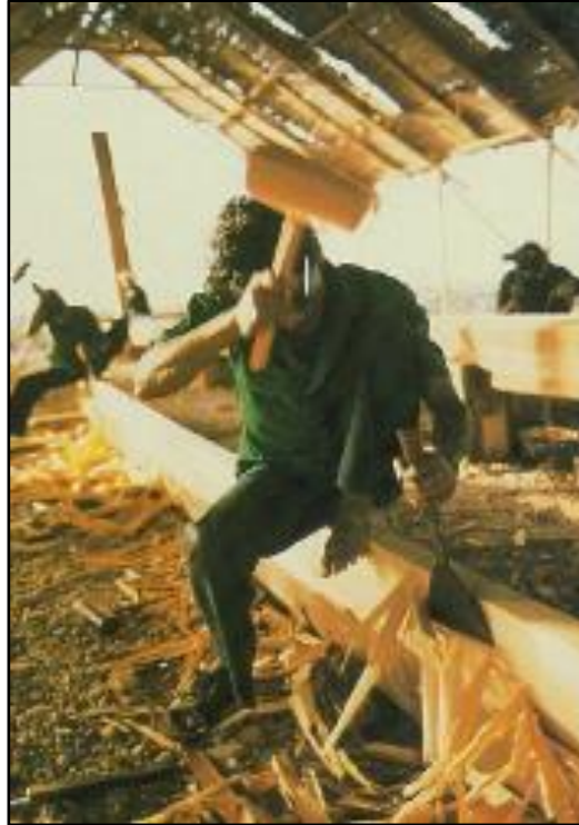
Shaping the timbers by hand chisel & hammer
